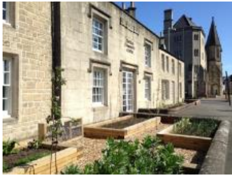
Front of Central Community Centre
